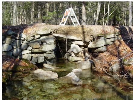
*Dry-laid stone box culvert on Gore Road, Warner, N. H., showing minor flood damage.
