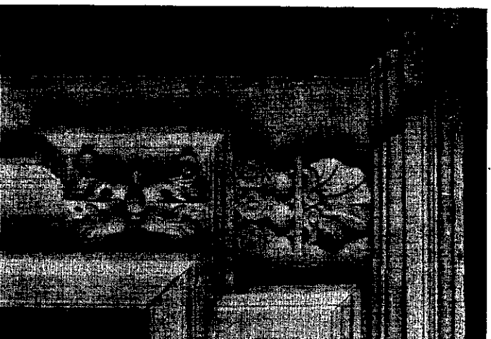
Fig. 5. Detail of mantelpiece, Colonel Joshua Wentworth House, Portsmouth, ca. 1770. (Historic American Buildings Survey; photograph by Clement Moran.)
