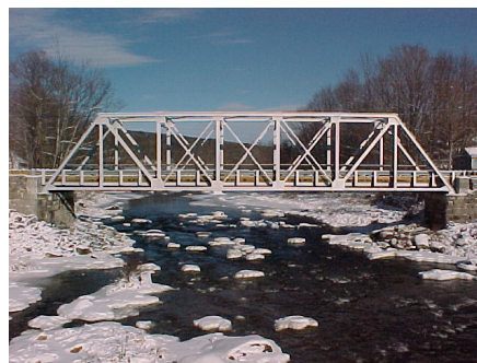
Patterson Hill Road Bridge, 1915, Henniker, NH (Photograph by James. L. Garvin)
