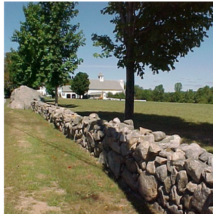
Stone wall along South Road Deerfield, NH (Photograph by James. L. Garvin)
