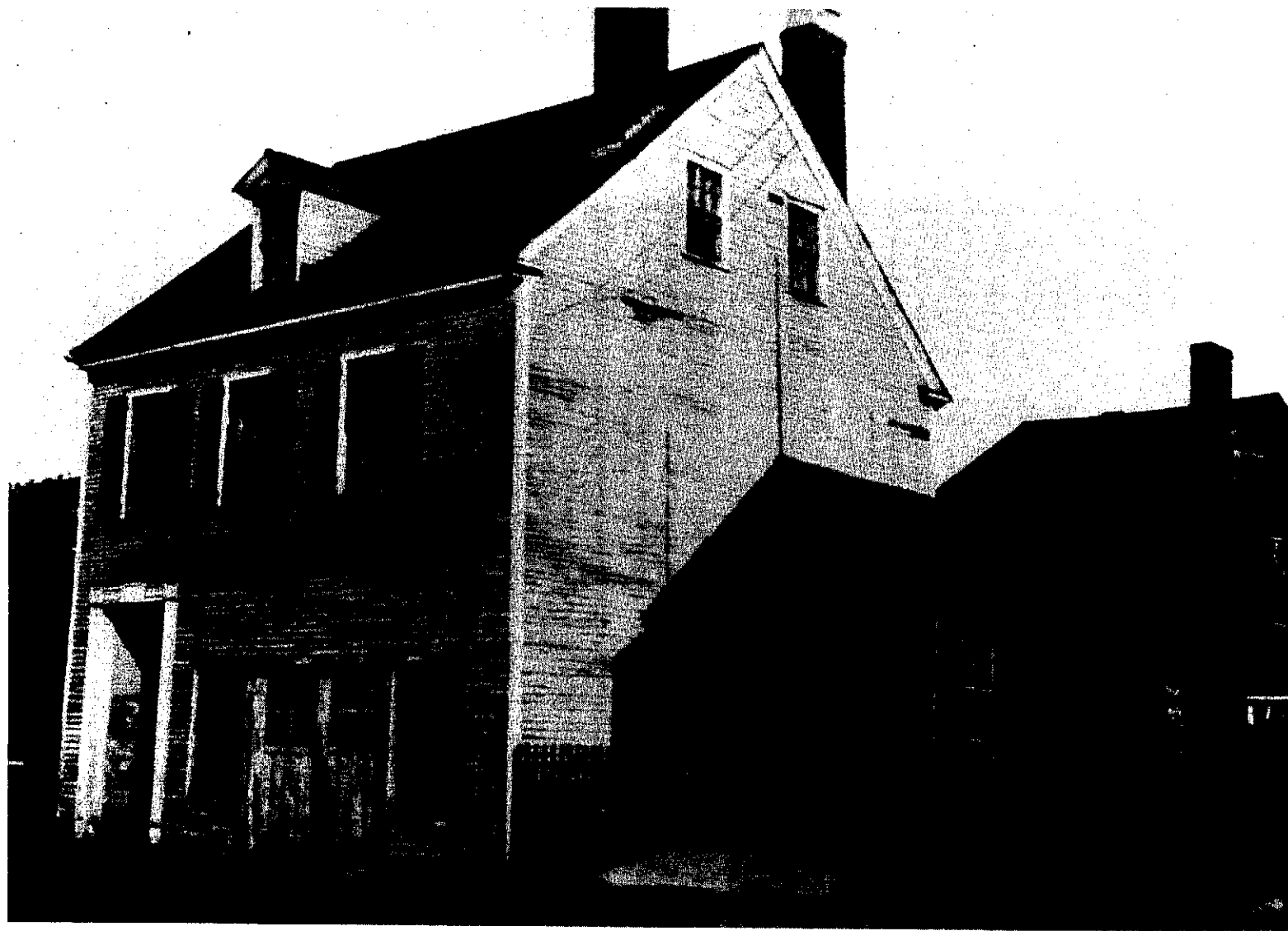
Remnant of the Old State House as it appeared on Court Street, Portsmouth, about 1935-38, with garage doors probably installed in the 1920s. Photograph by Arthur Harriman, courtesy Portsmouth Athenaeum Photograph Collections.
